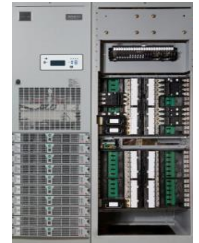
Electrical Distribution work
